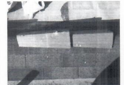
Fig. 2c. Lap Ridge Tile finished installation
